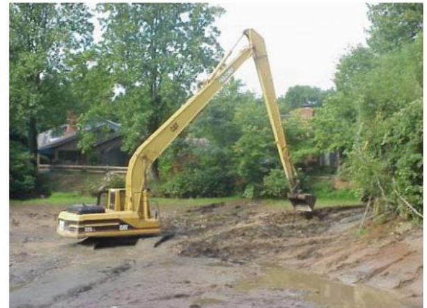
Muck removal and slope dressing by long reach backhoe
