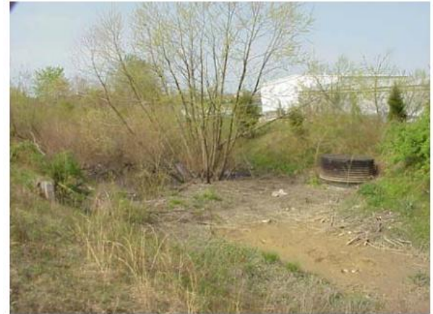
Sediment accumulation in a dry pond
